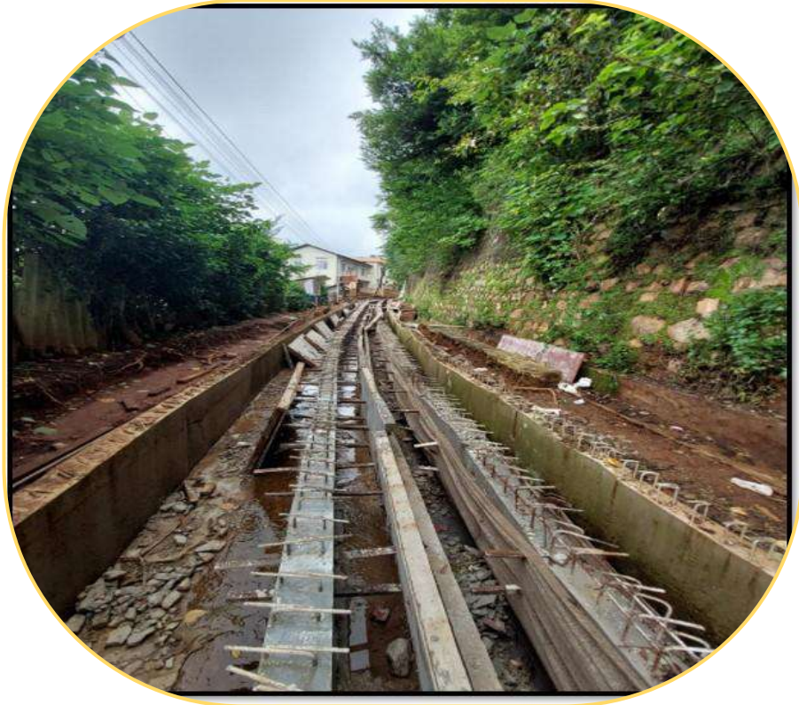
Construction of 6KM Smart Road
