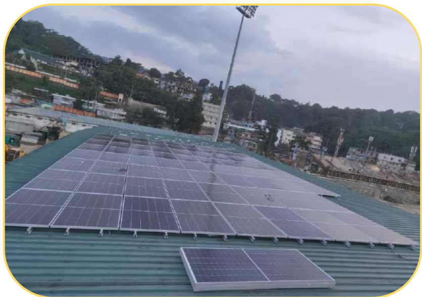
Installation of Solar at J.N Stadium
