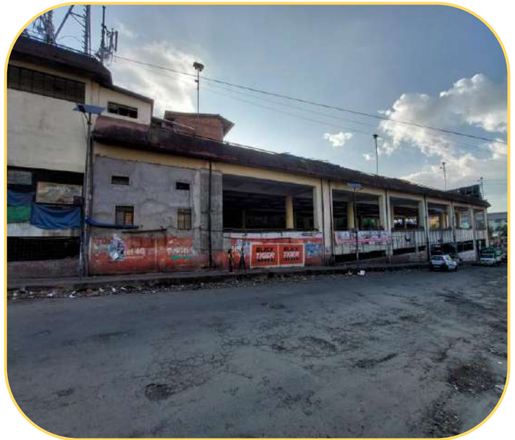
Retrofitting of Anjalee Parking Lot
