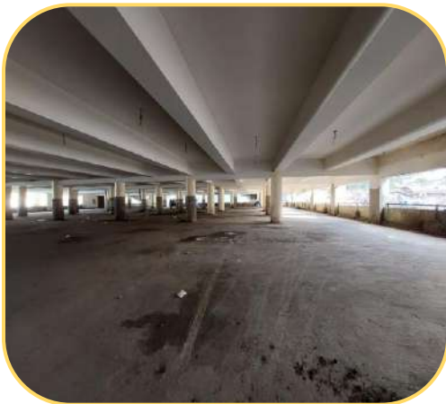
Retrofitting of Mawlonghat Parking Lot
