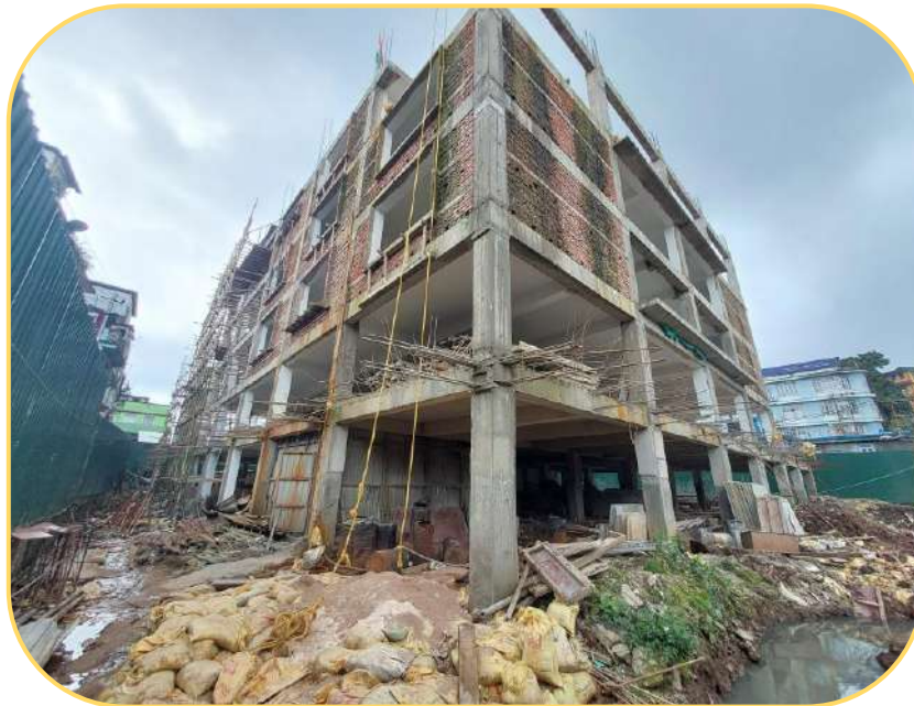
Construction of Laitumkhrah Commercial Complex
